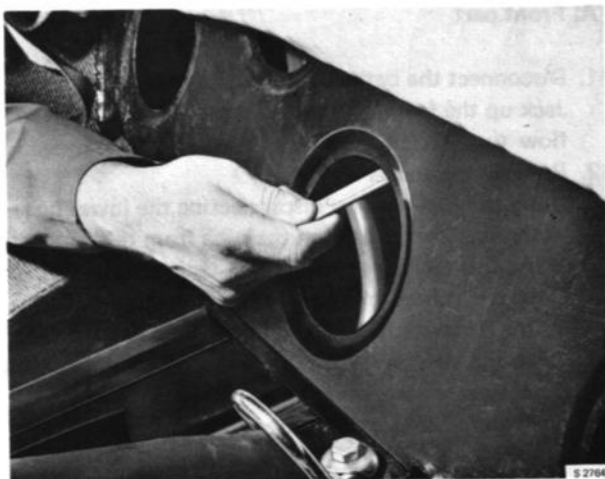
REMOVAL OF FUEL PIPE FROM TANK
