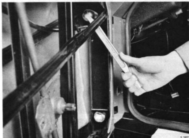
REMOVAL OF DOOR
