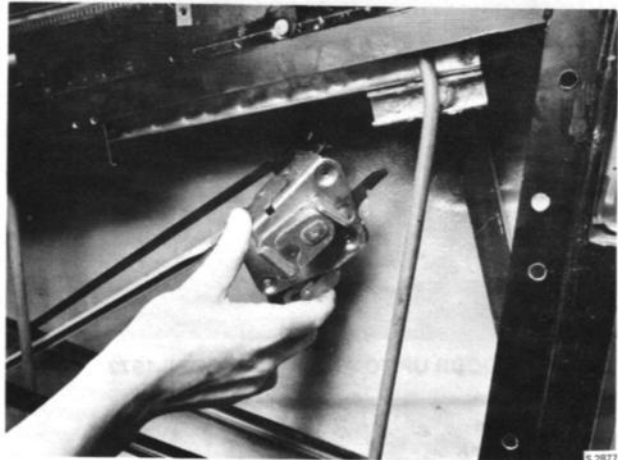
REMOVAL OF DOOR LOCK
